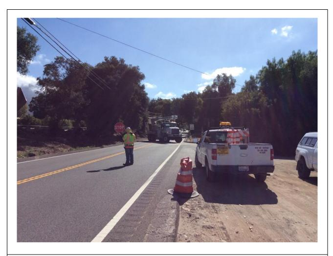
**Photo 6:** In accordance with APM TRANS-02, flaggers were present to maintain a safe travel corridor along Highway 76 during pole and equipment ingress to Pole Z115712 (TL682).
