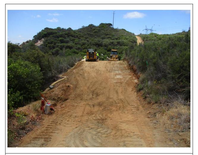
**Photo 3:** During grading of stringing site 5 (TL 6957), topsoil was salvaged and stockpiled for later use in restoration, in accordance with the Habitat Restoration Plan (MM BIO-4). Fiber rolls along the downslope perimeter of the work limits were effective in retaining sediment within the work limits and stockpiled topsoil was covered with jute mesh in accordance with the Erosion Control Plan and SWPPP (MM HYD-1).
